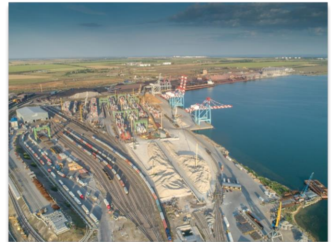
View on TIS Container terminal berth
